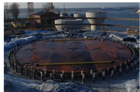
Fig. 9: Position of the mounting bolts in the concrete foundation and preparations for the measurement
