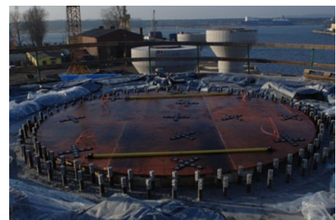
Fig. 9: Position of the mounting bolts in the concrete foundation and preparations for the measurement
